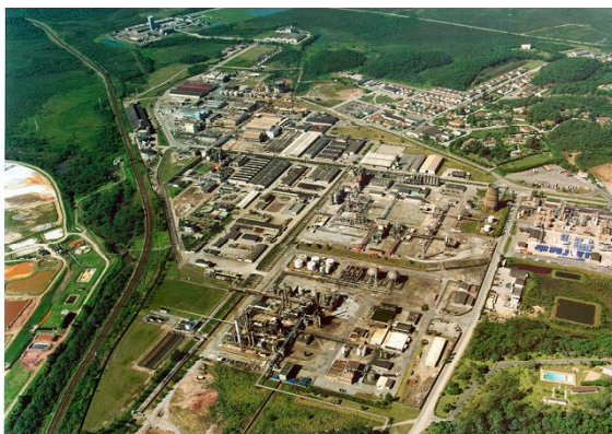
Solvay Indupa do Brazil, Elclor plant
